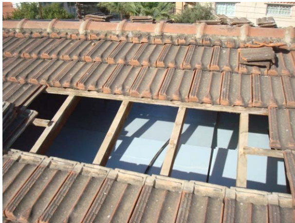
PP16 – Thermal Insulation of the roof
