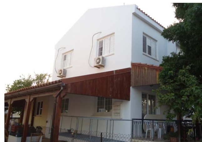
PP25 – After thermal plaster
