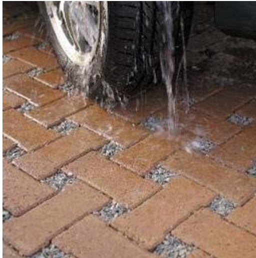
Figure 4. Permeable pavements – A SUDS measure
