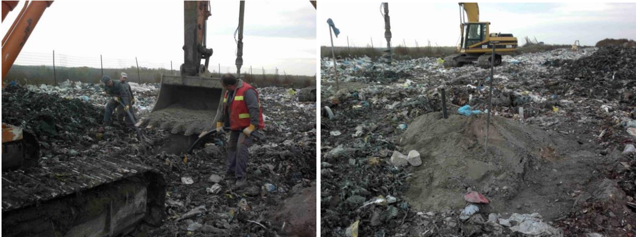
Figure 4. Construction of vertical heat exchanger wells
