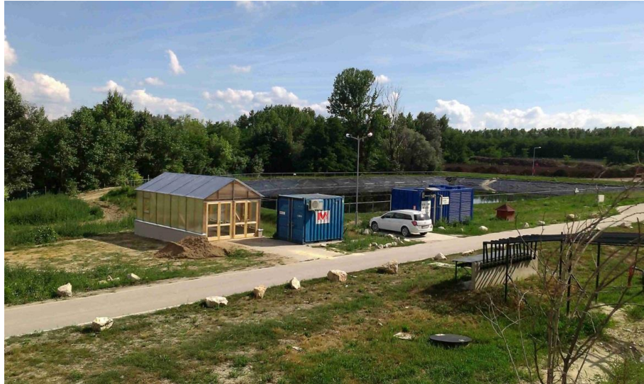
Figure 5. The built greenhouse, the container functioning as engine-house, and the leachate pond
