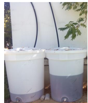
Figure 2. Deposit to collect leaching from green roofs
