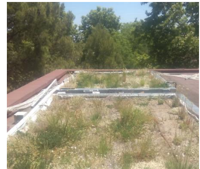
Figure 1. Piece of grounds of the Extensive Green Roof in University of Córdoba
