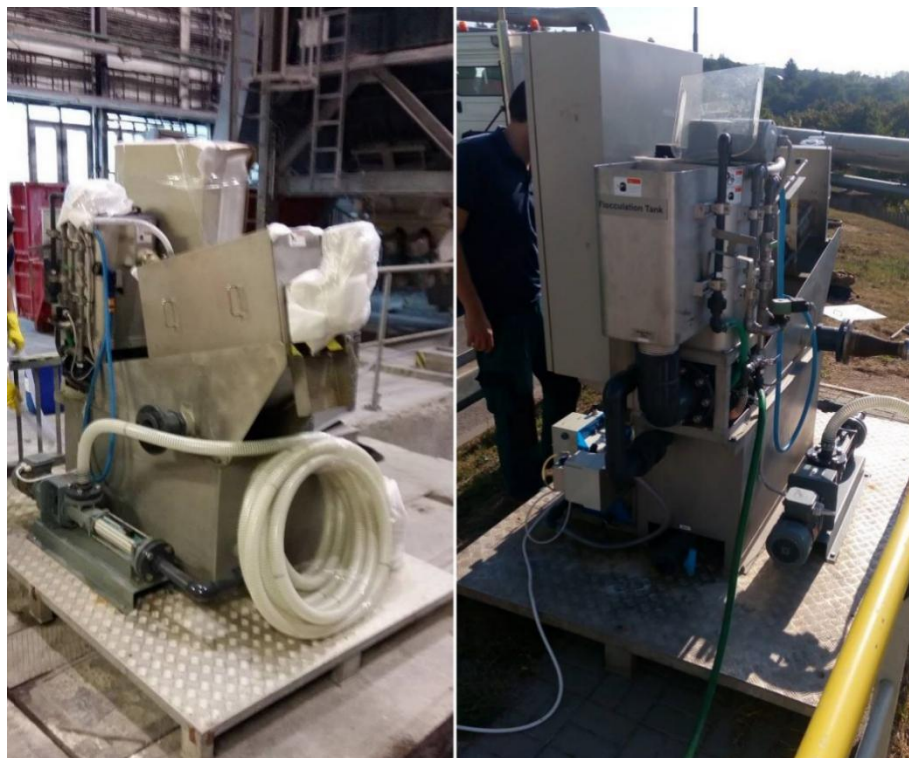
Figure 2. Pilot testing in real condition, left: bottom ash tank, right: retention tank.
