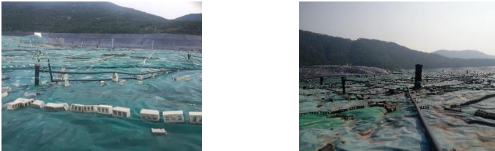
Fig. 2. On-site pictures of vertical shaft collection system in refuse landfill of Fujian province
