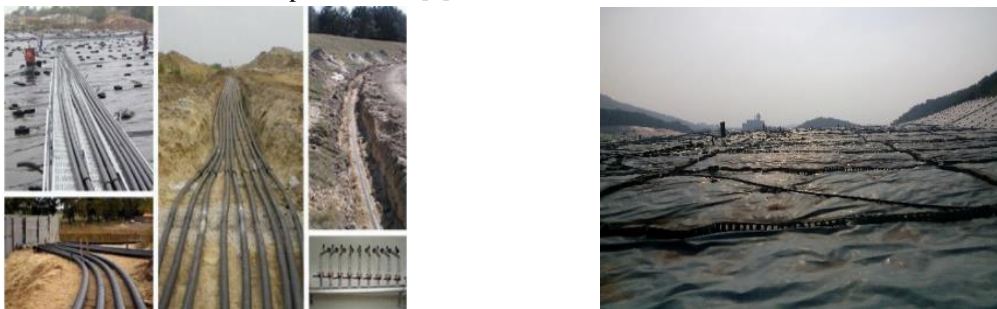
Fig.1. On-site pictures of efficient collection system of GHG in refuse landfill of Liaoning province.
