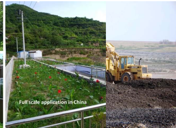
After dewatering Alum sludge can be landfilled or used in constructed wetland (AICW)
