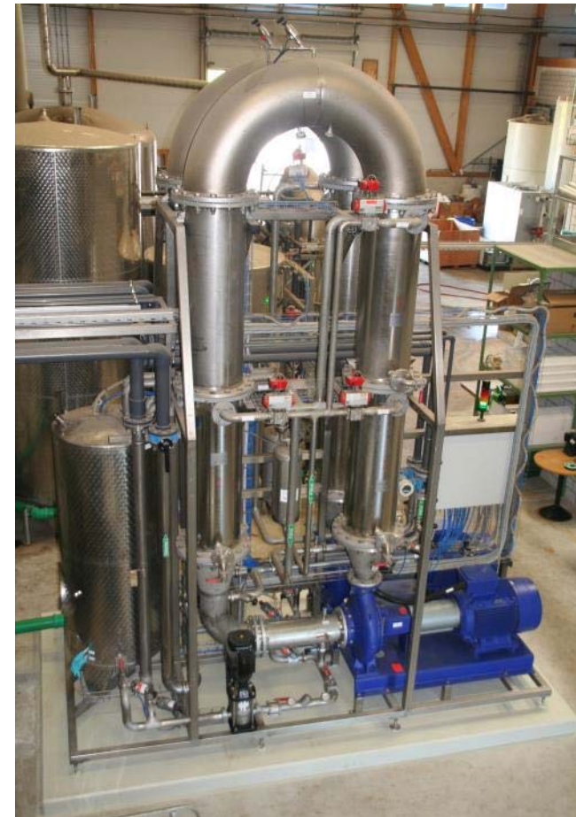
Fig. 3: Ultrafiltration plant Inwil- Switzerland
