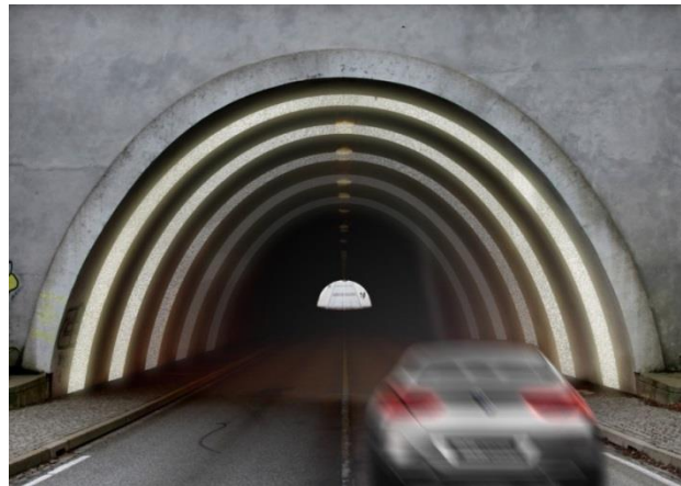
Figure 8. BlingConcrete™ in tunnel [43]
