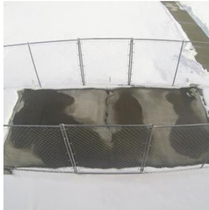
Figure 9. Electronically conductive concrete [49]
