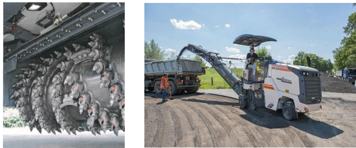
Figure 2. Scraping of old bituminous surface layer [29]
