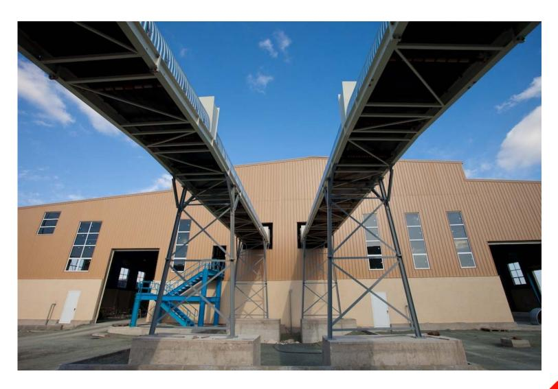
After the bag openers the waste stream is transported through conveyor belts inside the Mechanical Separation Hall, where all sorting-recovering processes take place.
