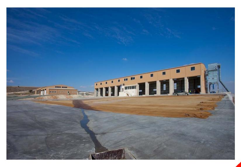
All garbage trucks are directed to the weighing station, where they are automatically recorded, weighed and subsequently directed to the Reception Hall. The Reception facility is capable of accommodating the simultaneous unloading of 8 trucks. All 8 unloading positions (doors) are equipped with a automatization which supports the complete unloading process (truck approaching, unloading and departure).
