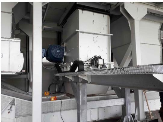
**Figure 5.** New hammer mill as pre-shredder
