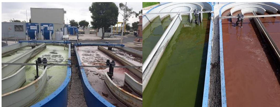
Figure 1. Incover demonstration ponds. On the left side of the pictures it is shown the initial stage of HRAP retrofitting (green color from algae). On the right side of the pictures it is shown an already retrofitted HRAP converted into a PPBpond and enriched in PHA-accumulating phototrophic purple bacteria (red-brown color).
