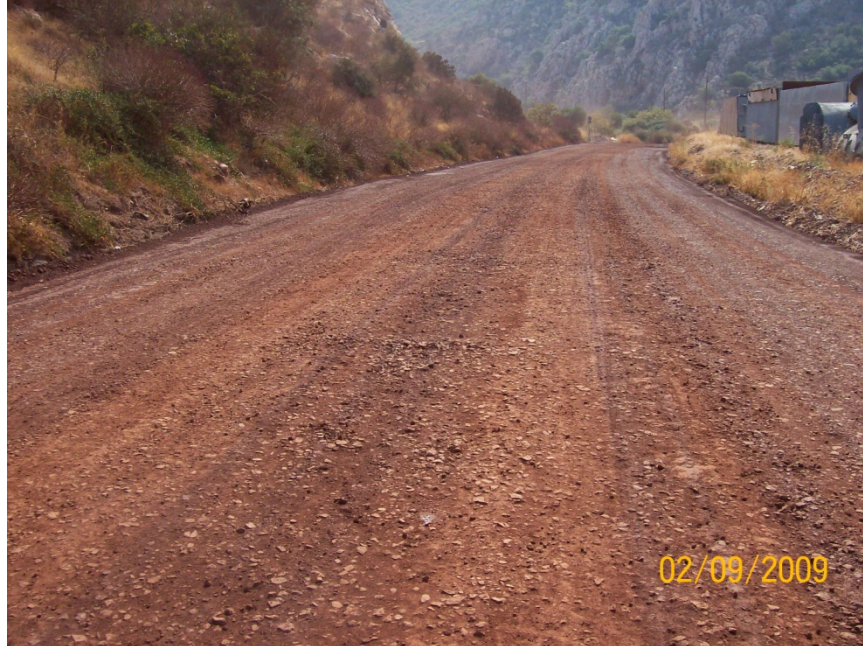
Fig. : Local road constructed from bauxite residue
