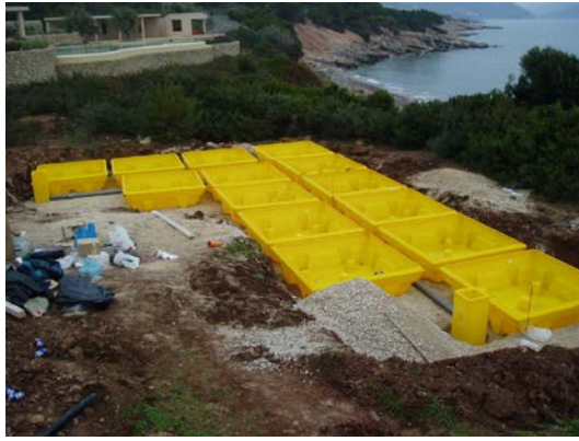
Figure 8. Construction standardized biological operation unit 50 PE [7.7]
