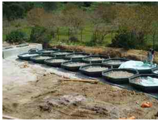
Figure 11. The basins are filled with graded aggregate inert, and placed a membrane preferably geotextile [7.7]
