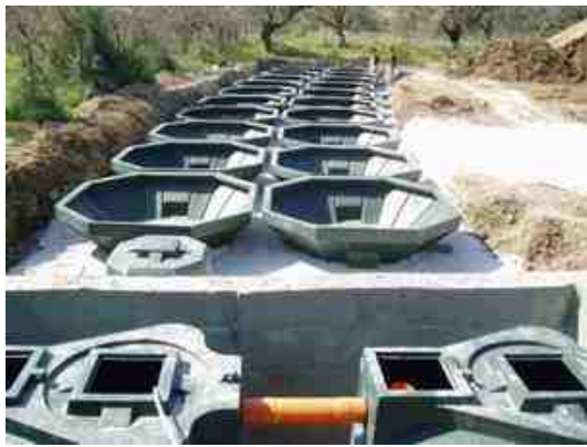
Figure 10. Installing a standard unit 50 P.E. Porto-Cheli.- Greece [7.7]
