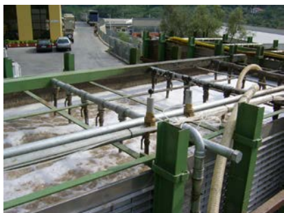
Fig.3. WWTP ((courtesy of GOST solutions)
