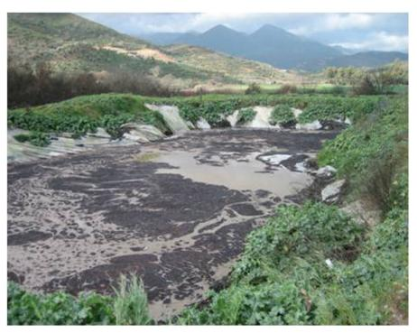
Evaporation ponds are widely used worldwide despite the fact that in some cases only waste volume is reduced and serious problems might occur due to leakage of wastewater to soil and/or groundwater
