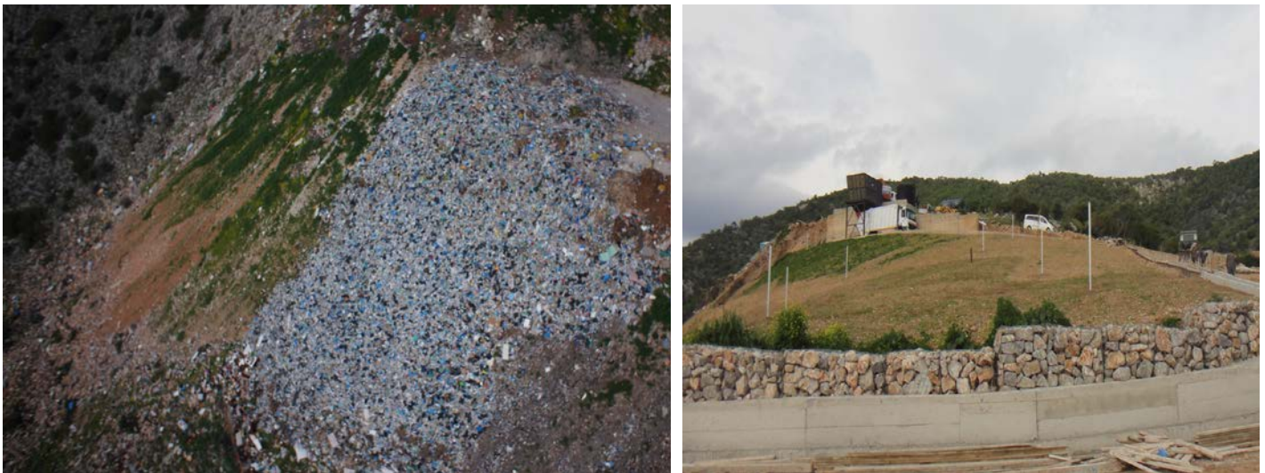
Dumping site before and after restoration 13
