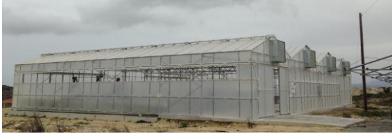
Picture 1. General view of the Solar drying greenhouse unit (Fertenergy)
