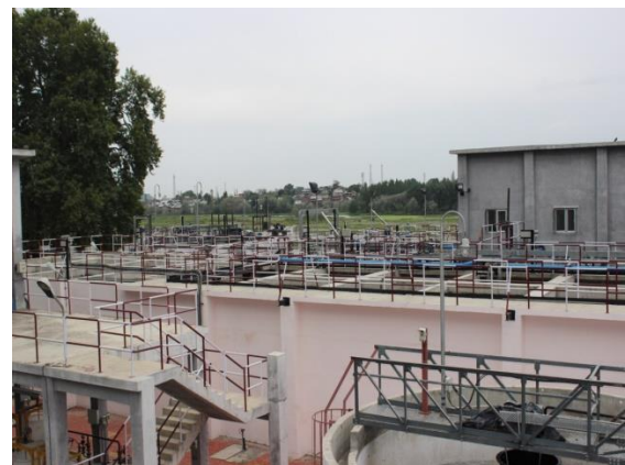
Picture 2: H-Batch system for a capacity of 5,400 m 3 /d (40,000 PE) in Srinagar/India
