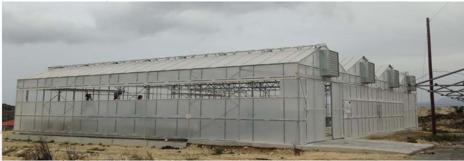
Picture 3. General view of the Solar drying greenhouse unit
