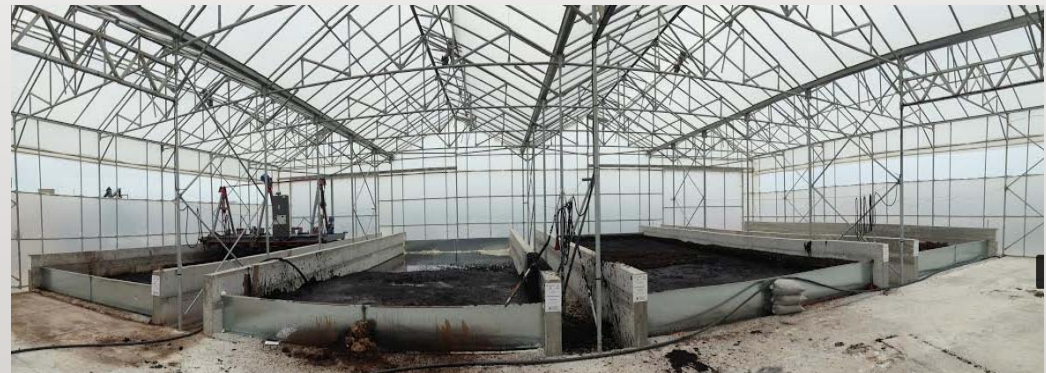
Picture 4. Inside view of the Solar drying greenhouse unit (four corridors)
