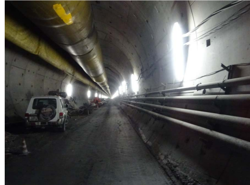
Second Tunnel at Frejus under construction
