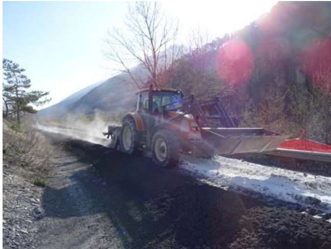
Lime stabilization of sludge for drying
