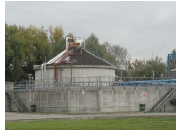
2000 m 3 anaerobic digester CSTR
