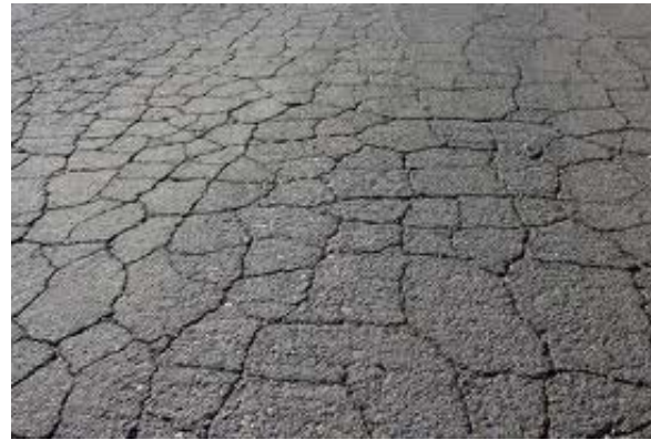
Intermediate T Fatigue Cracking
