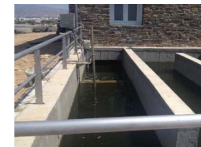
Chlorination & dechlorination stages
