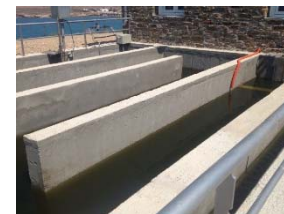
Chlorination & dechlorination stages
