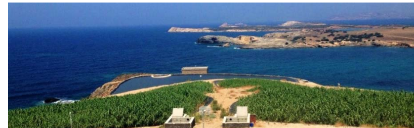
The two stages of CWs & the stabilization pond
