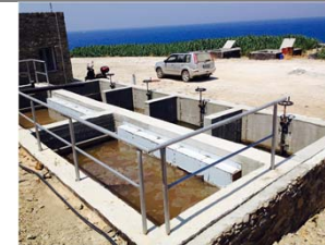
Imhoff tanks for WW sedimentation
