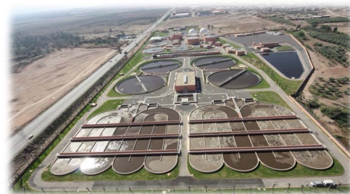
WWTP of Marrakech
