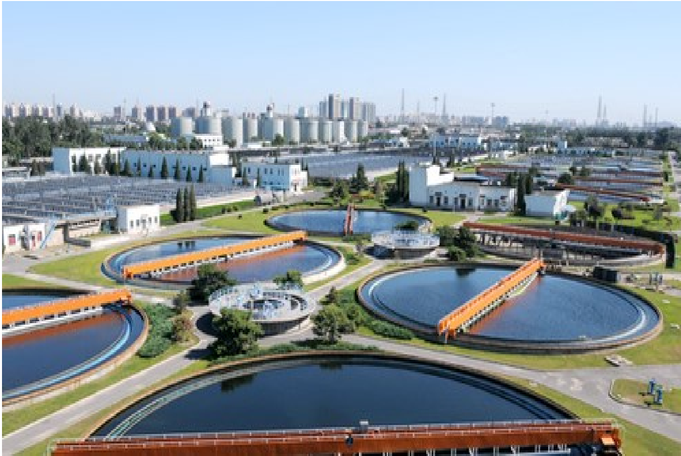
Gaobeidian WWTP in Beijing, Capacity: 1 million m 3 /d in 1999
