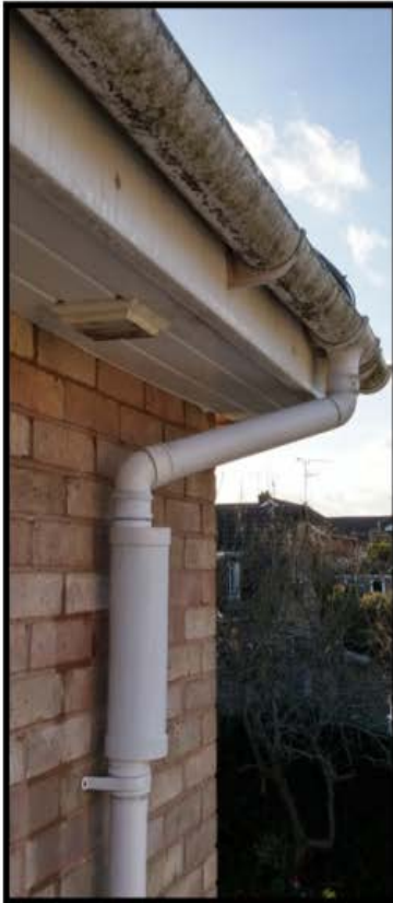
A) Chamber connected to downpipe
