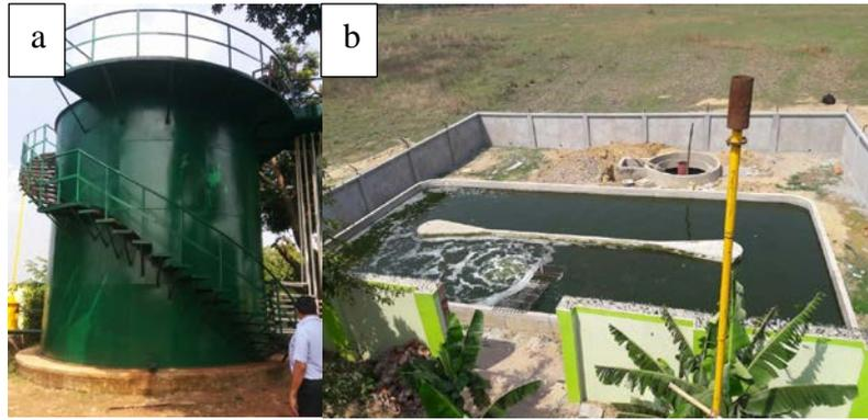
Figure 1: (a) UASB reactor, (b) HRAP
