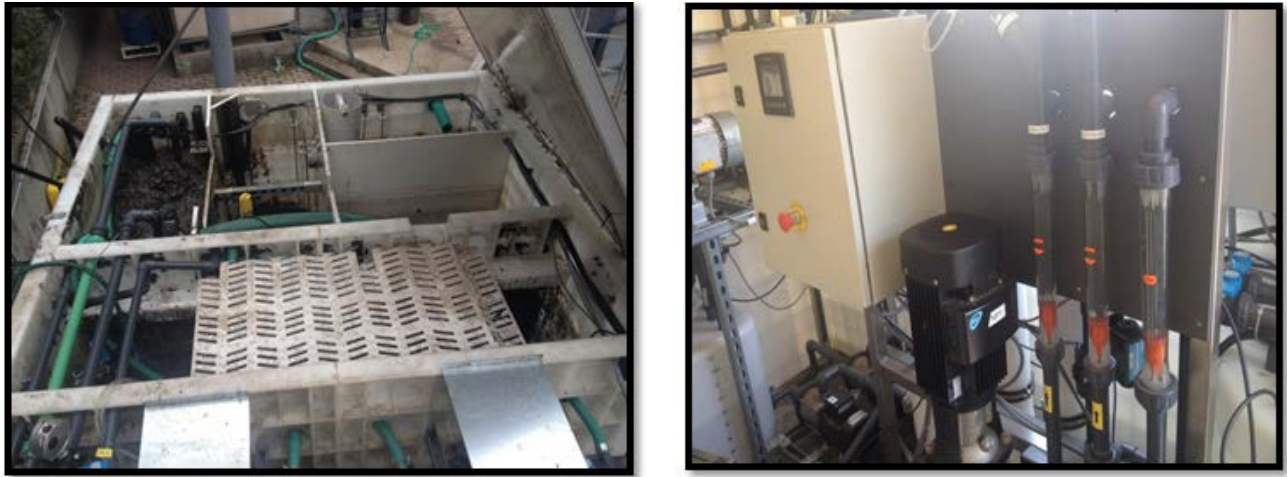
Fig. 2. Presentation of DESSIN's pilot plant. The left photograph depicts the compact unit containing (from the left to the right) the MBR, aeration, anoxic and equalization tanks, while the right one shows the Reverse Osmosis.
