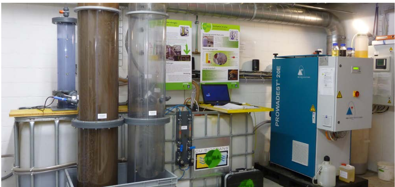
Figure 3. The VUNA moving-bed biofilm reactor stabilises the urine, before it is concentrated in an industrial distiller to produce a liquid fertiliser. A similar reactor is installed in the Water Hub.
