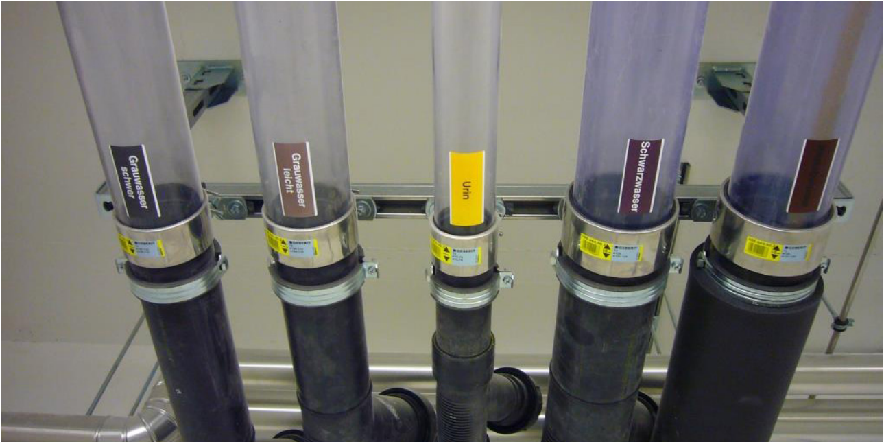
Figure 1. Five different pipes convey the various wastewater types to the Water Hub: light and heavy greywater, urine, brownwater, and mixed wastewater. Not on the picture: rainwater pipe.
