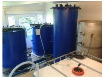
**Figure 1:** Decentralised anaerobic pilot plant for producing domestic service water out of domestic wastewater. The plant is built up in the communal sewage plant of Erlangen, Germany. The plant is integrated in two standard office containers that are connected to one room cell with a total area of 28 m<sup>2</sup> and a ceiling height of 2.50 m.
