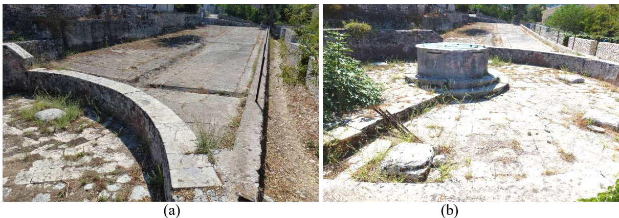
Figure 3. Agioi Anargyroi cistern. a. The western runoff surface. b. The central-original(?) runoff surface, the orifice with the raised access corridor and the the intake spouts covered with slabs . On the orifice is visible the inscription in dark gray colour.
