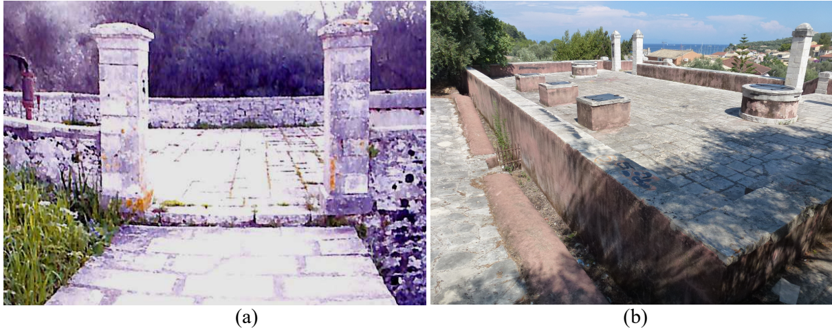
Figure 2. a. Main view of the Vlacherena circular rainwater cistern (Doikas, 2005). b. View of the paved runoff surface of Ag. Apostoloi cistern and the round orifices of the min reservoir, as well as the cubic openings of the auxiliary tank
