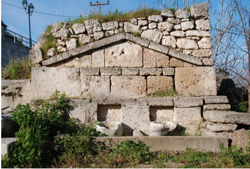
Figure 12. The masonry at Murat Ağa fountain's façade.
