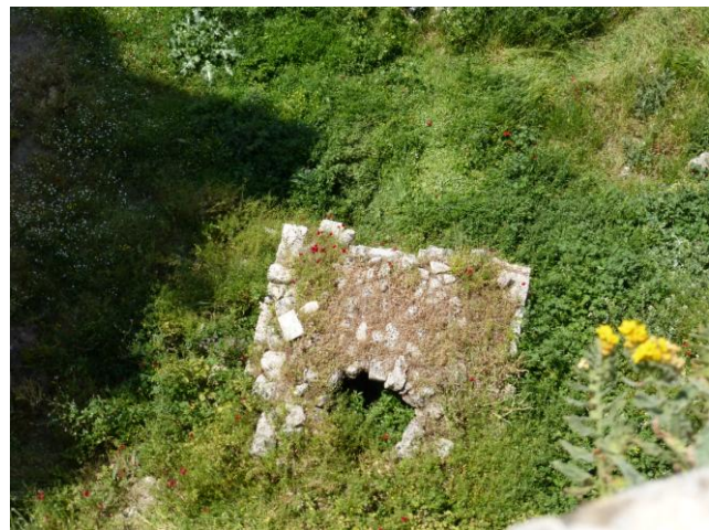
Figure 18. The low barrel vault covering the water tank.
