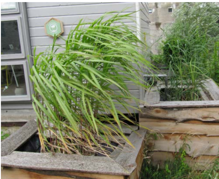
Figure 2. Individual biofilter (2 tanks) for grey water treatment.
