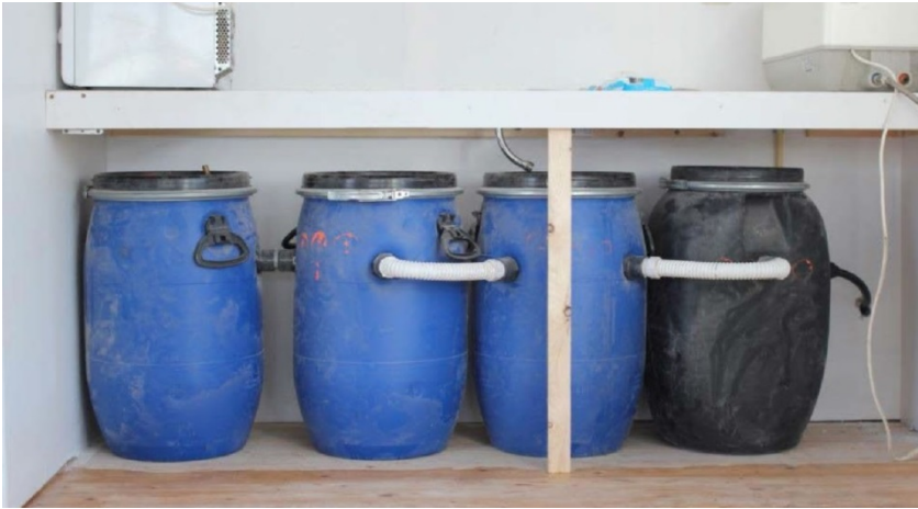
Figure 3. Settling drums (60 litres per drum) under the sink of a boat.
