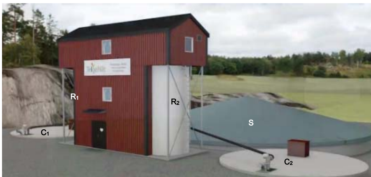
Figure 1. The treatment plant sanitising black water with a combination of auto-thermal aerobic digestion and ammonia treatment, showing the two 32 m 3 ATAD reactors (R) (built in), the two below surface, insulated 200 m 3 collection basins (C) and the covered, above ground 1500 m 3 covered post-treatment storage basin (S) ( www.telge.se/vatten-avlopp/kretsloppsanlaggning ).
