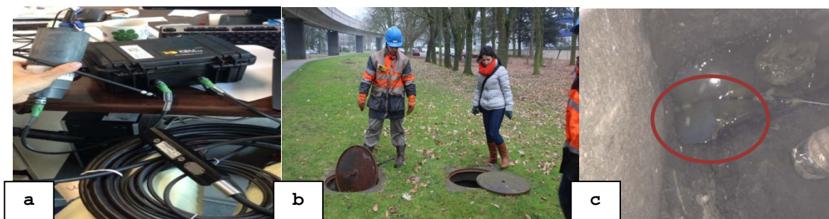
Figure 9: Flow meter installation (a) flowmeter, battery and data logger (b) installation step, (c) installed sensor in the manhole
