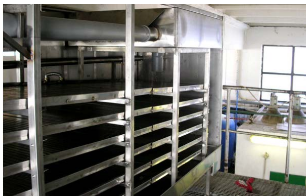
Figure 8. An example of a desk heat exchanger for heat recycling from grey water.
