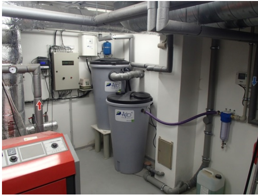
Figure 7. An example of devices for grey water recycling – treatment plant for grey water and spiral heat exchanger
