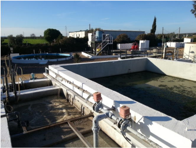
Figure 2. Picture of the activated sludge system-30 m 3 /day at CENTA (Seville)
