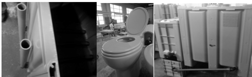
Figure 1. Main features of UDDT systems: (from left to right) air admission into composting chamber; ceramic toilet and layered toilet seat; urine reservoir and composting box
