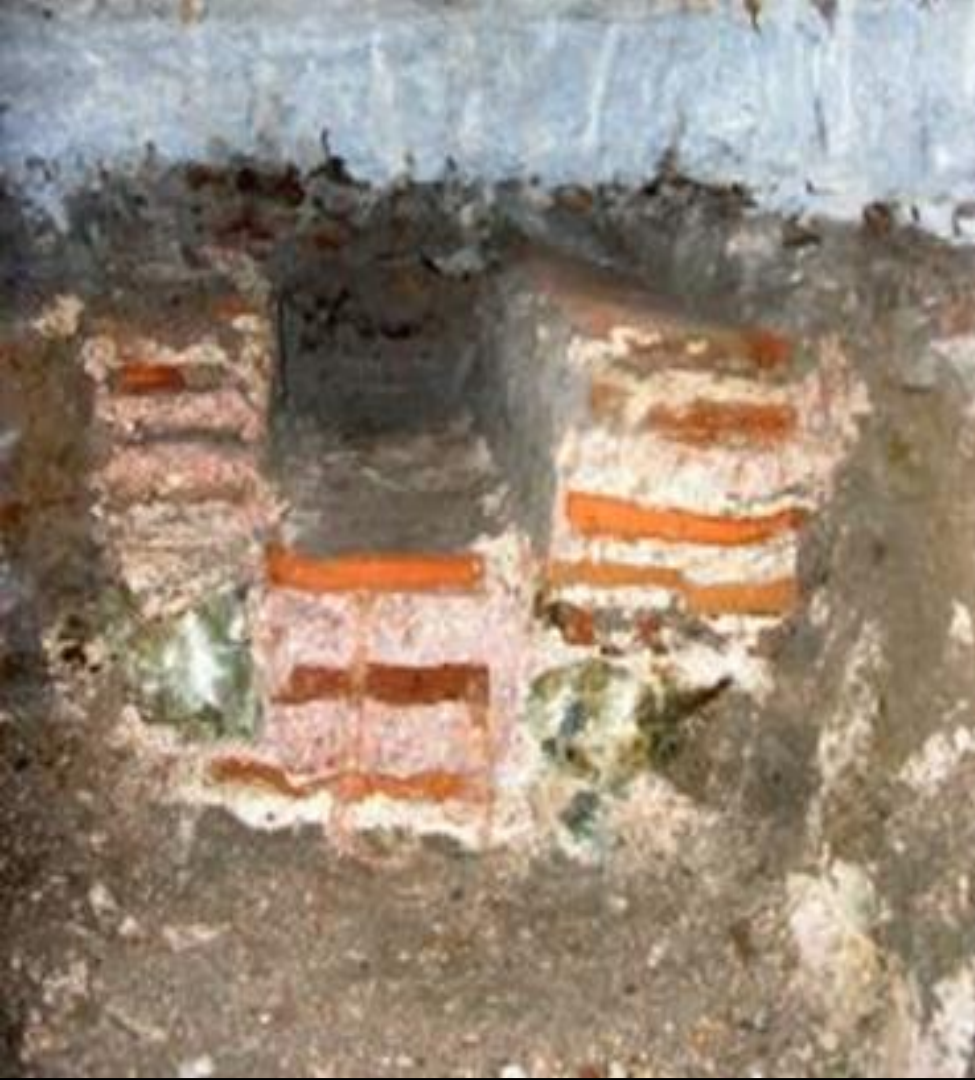
Roman time sewers in Thessaloniki : (a) closed to walls and (b) central sewer covered with stone-build apsis
