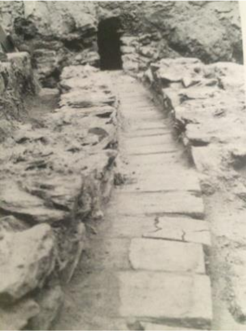
Stone-build sewers of Byzantine time (6 th c.): (a) in Pastier road and (b) in Egnatia road.
