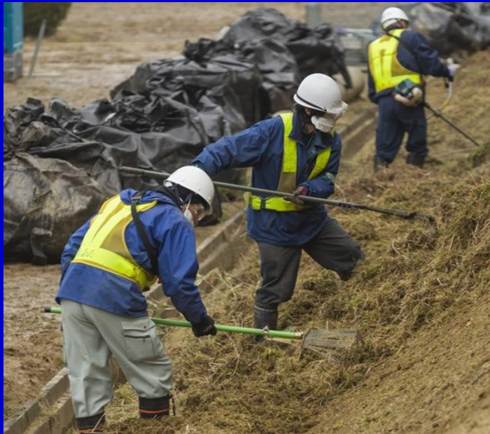
Stripping work of contaminated soil and leaves
