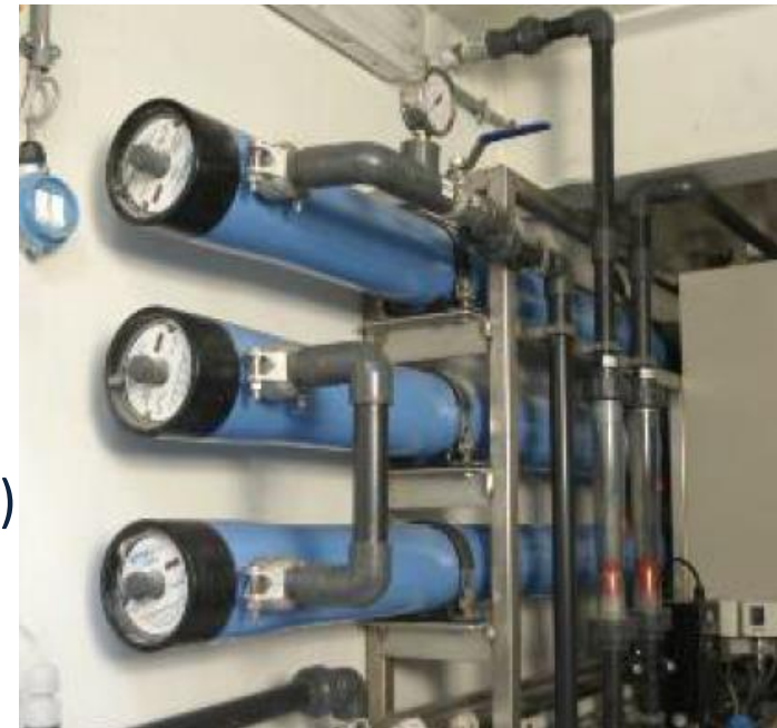
Figure: Pressure vessels containing the RO membranes
