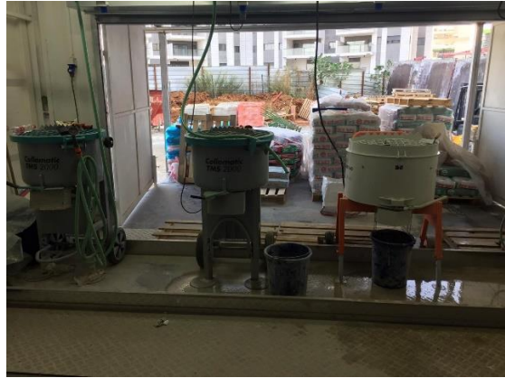
Fig.1 The centralized mixing and supply of bulk materials in company A
