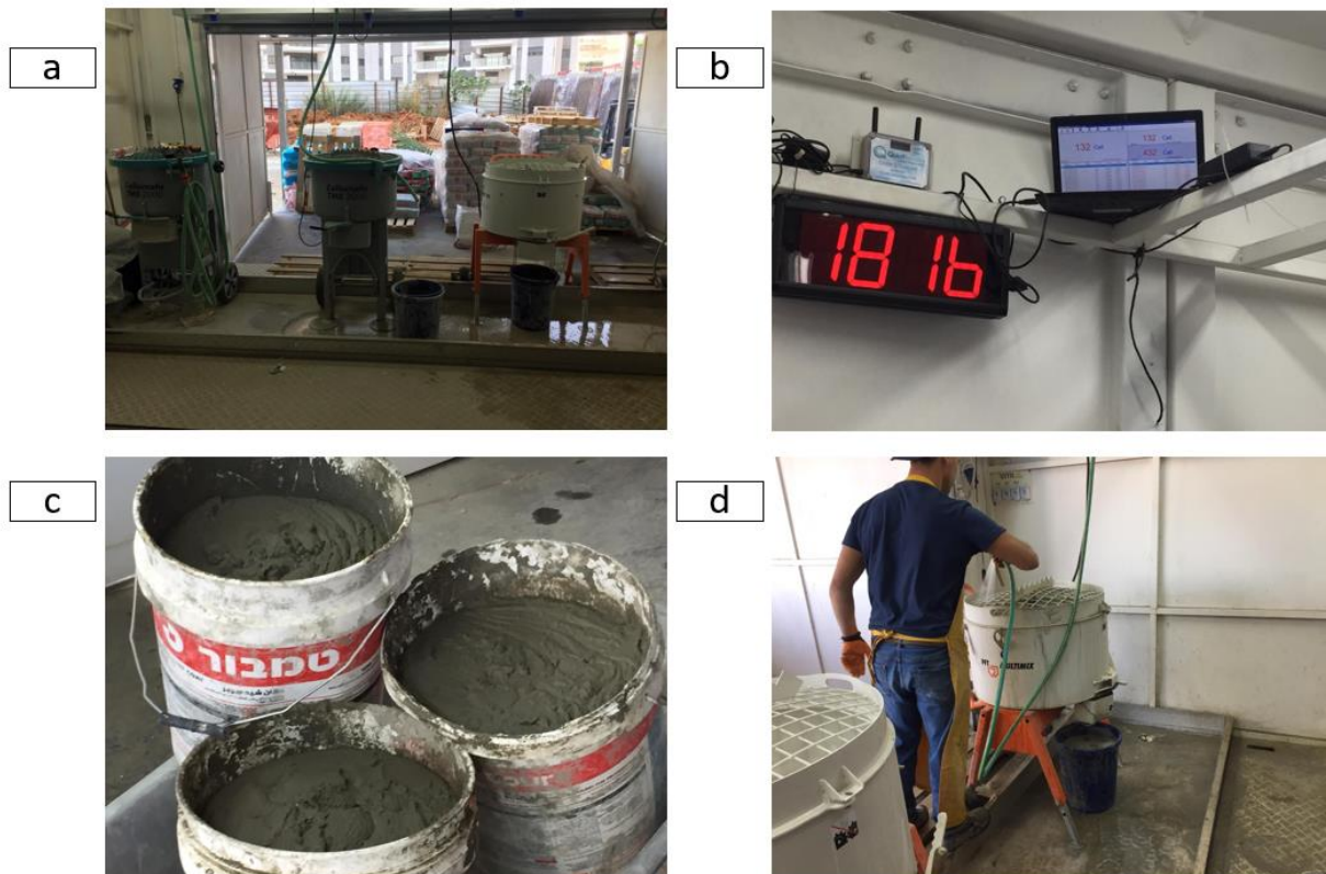
Fig. 3 Illustrations of the centralized mixing; a) scope of the station; b) Kanban tool; c) the ready-mix mortar; d) cleaning the mixer
