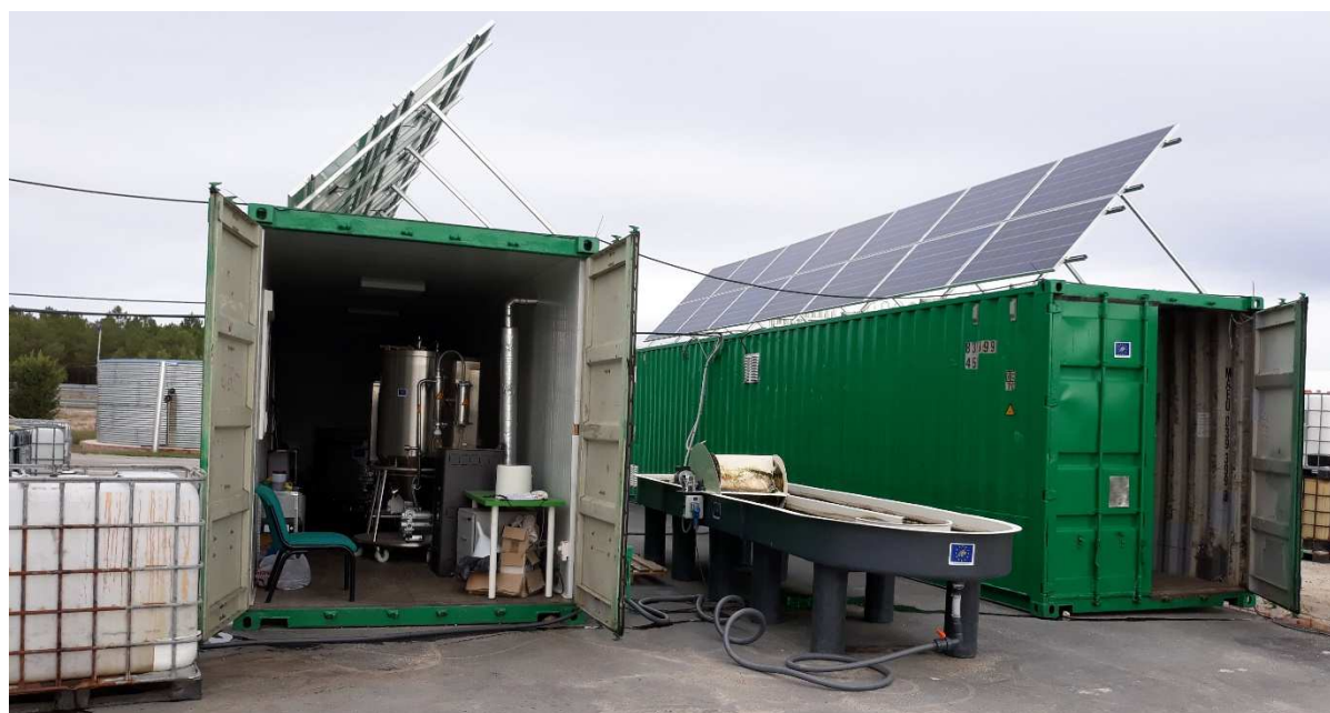
Figure 1. Pilot plant for the treatment of wastewater with heterotrophic microalgae.
