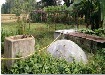
Figure 1: Defunct household biogas digester in Napaam
