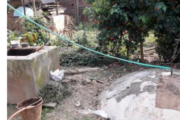
Figure 2: Functioning household biogas digester in Amlighat
