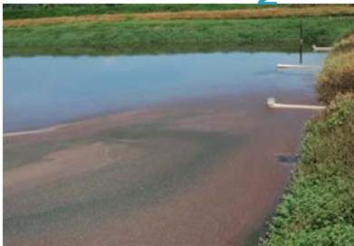
Waste water treatment
